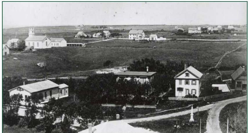
View of Chatham in 1886 from the belfry of the Methodist Church. In this view we can see the Old Baptist Church, now the Masonic Building on Old Harbor Road; further up is the Old Alms House (Poor Farm), now the parking lot of Holy Redeemer Catholic Church, and further still the Granville Seminary where Bank of America is now located. In the foreground in the center is what was Washington Hall, home of J. Howard Nickerson, and next to it the former parsonage of the Congregational Church, now an antique shop. Also in the foreground is the Soldier’s Monument with its old original pump.
