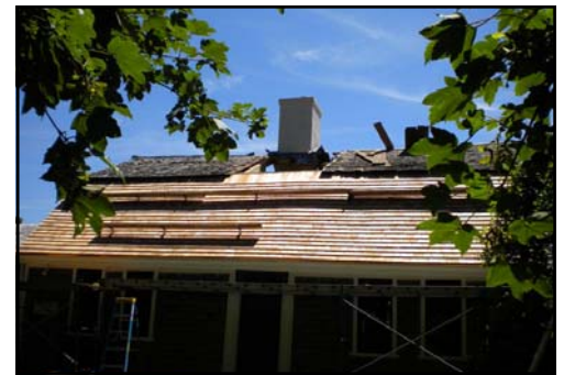
New roof shingles replacing the old ones
