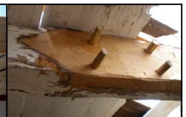
new scarf joint
